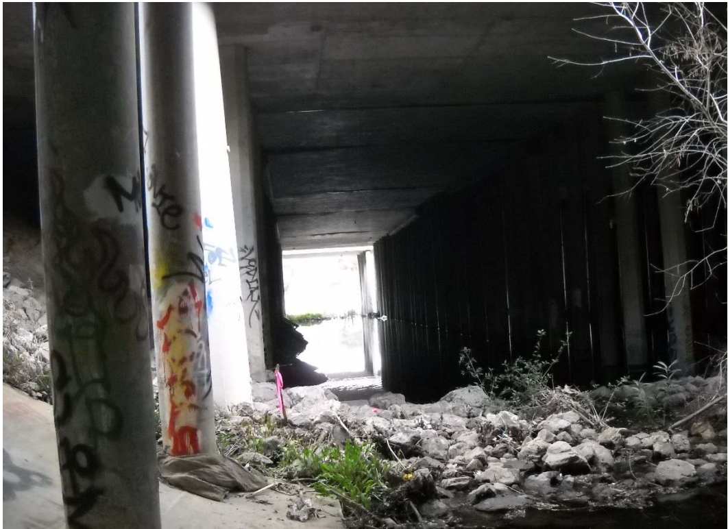
UPSTREAM & DOWNSTREAM EXTENT OF REACH No. 35, BENEATH U.S. HWY 101 BRIDGE HEC-RAS RIVER STATION 25+35, DOWNSTREAM DIRECTION
