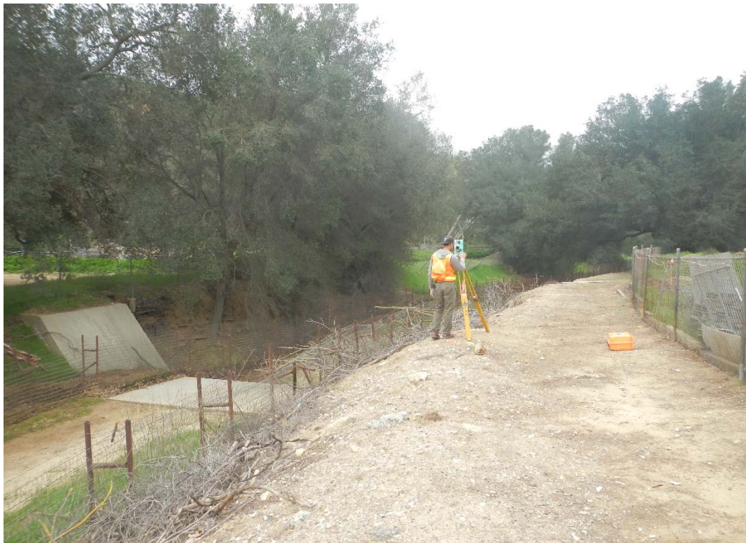
HEC-RAS RIVER STATION 12+33, DOWNSTREAM DIRECTION
