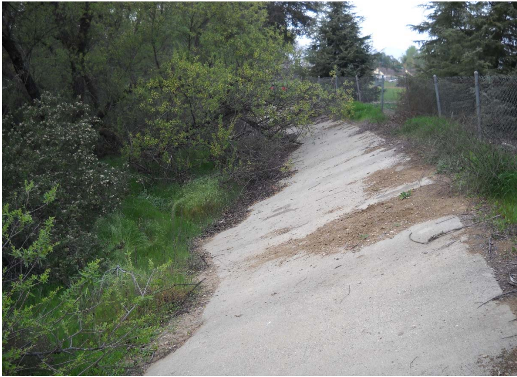
HEC-RAS RIVER STATION 35+52, LEFT BANK, UPSTREAM DIRECTION
