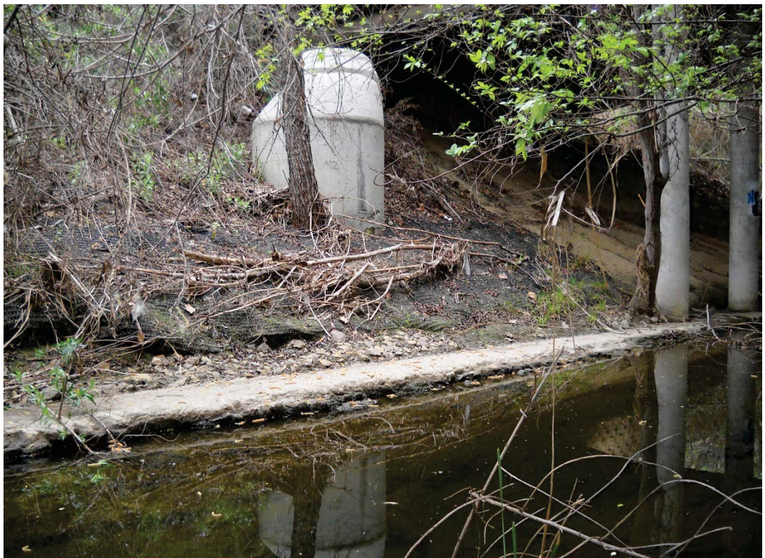
Figure 6-6. Stormwater Access at Oak Creek Lane Bridge
