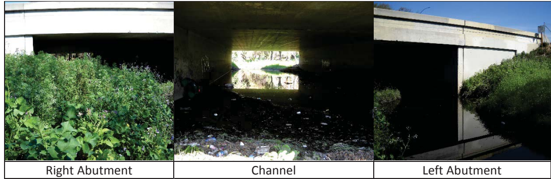
Figure 2-2. Artesia Blvd Bridge
