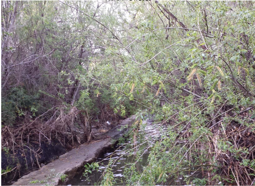
HEC-RAS RIVER STATION 30+48, UPSTREAM DIRECTION
