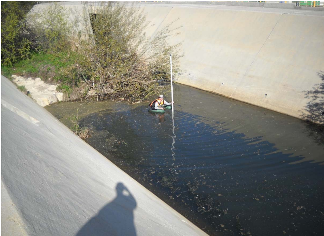
30 FT. UPSTREAM OF HEC-RAS RIVER STATION 63+70, UPSTREAM DIRECTION
