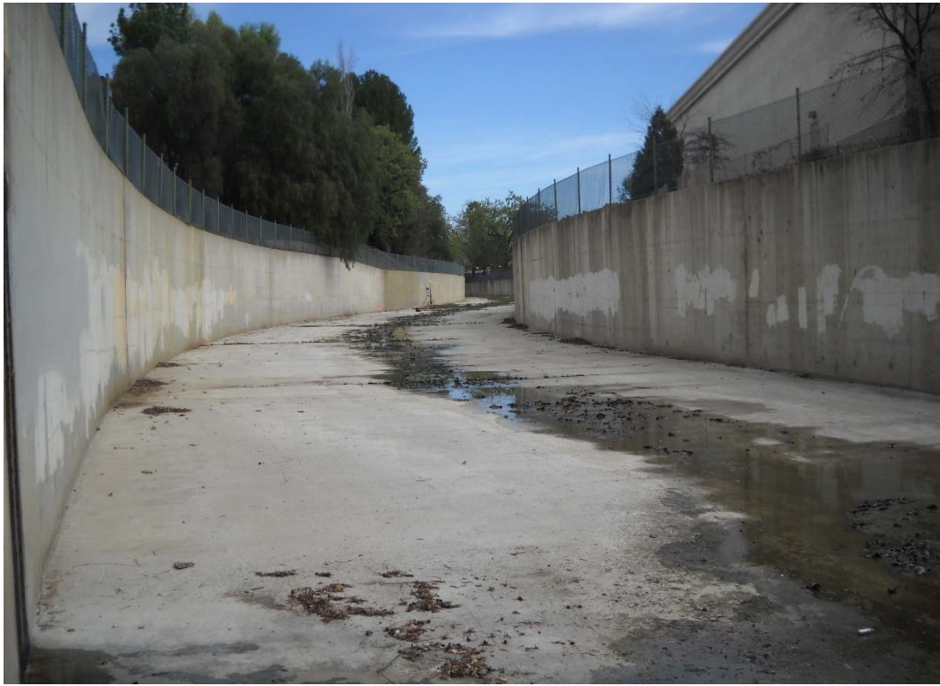
HEC-RAS RIVER STATION 00+16, UPSTREAM DIRECTION
