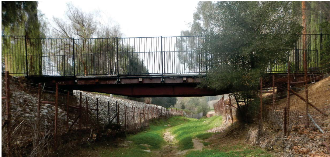
Figure 5-2. Stokes Canyon Channel Residential Access Bridge
