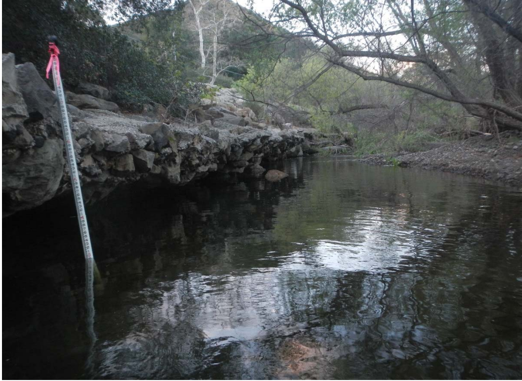
HEC-RAS RIVER STATION 15+39, UPSTREAM DIRECTION
