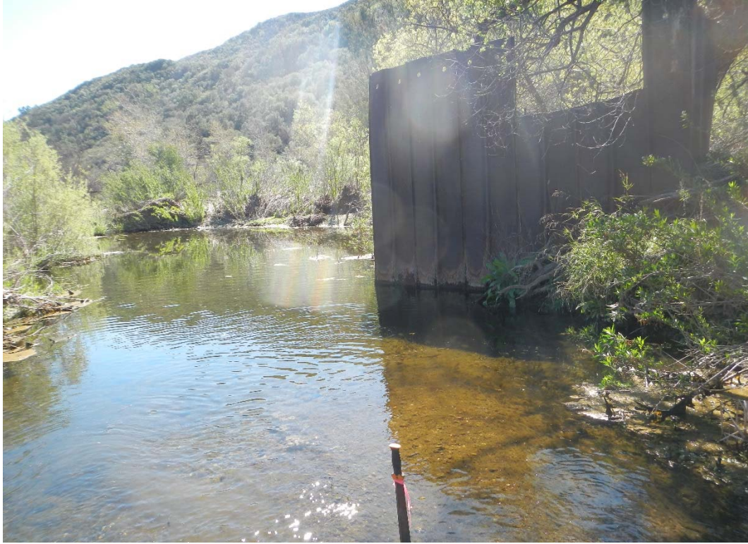
HEC-RAS RIVER STATION 7+67, DOWNSTREAM DIRECTION
