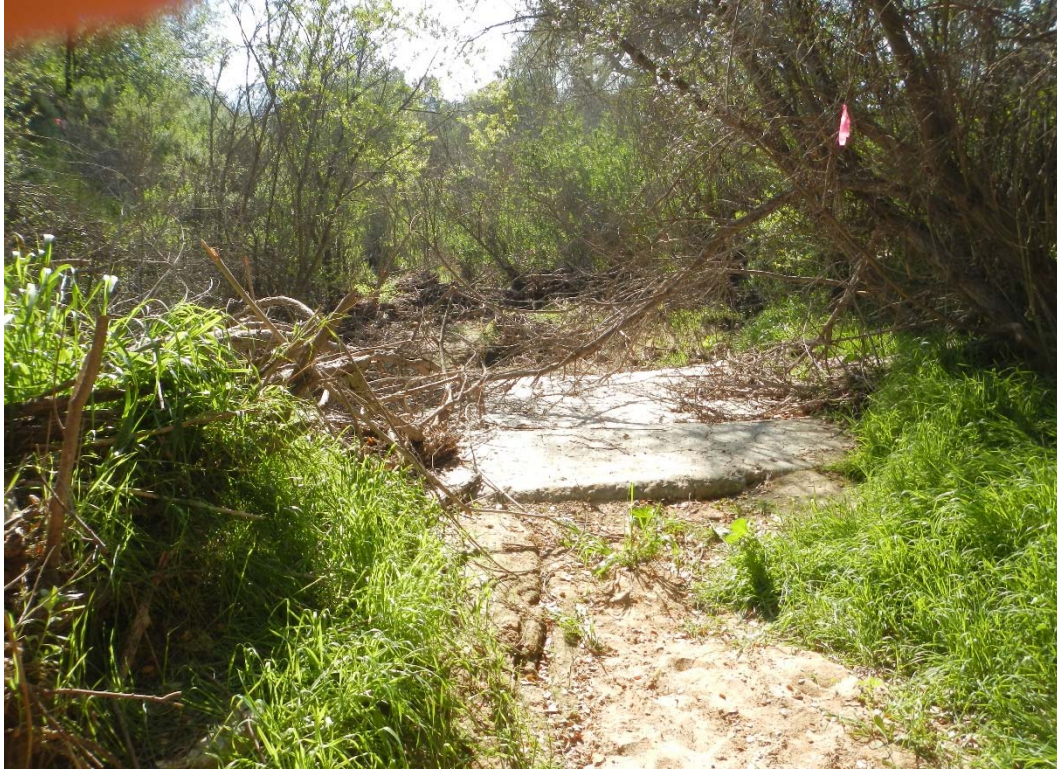
HEC-RAS RIVER STATION 7+00, DOWNSTREAM DIRECTION
