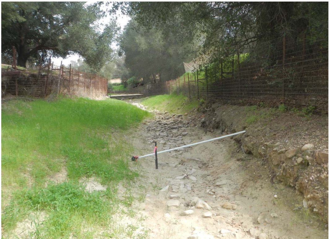
HEC-RAS RIVER STATION 10+50, UPSTREAM DIRECTION
