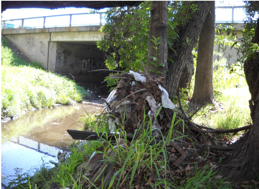
HEC-RAS RIVER STATION 7+74, DOWNSTREAM DIRECTION
