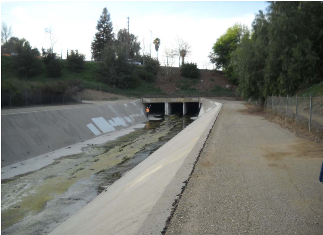
56 FT. UPSTREAM OF HEC-RAS RIVER STATION 39+69, UPSTREAM DIRECTION KANAN RD. CULVERT (UPSTREAM OF REACH NO. 34)
