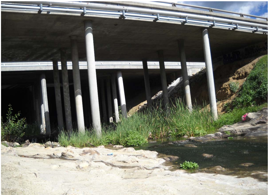
HEC-RAS RIVER STATION 22+42, UPSTREAM DIRECTION (ROADSIDE DR. & HWY 101 BRIDGES)
