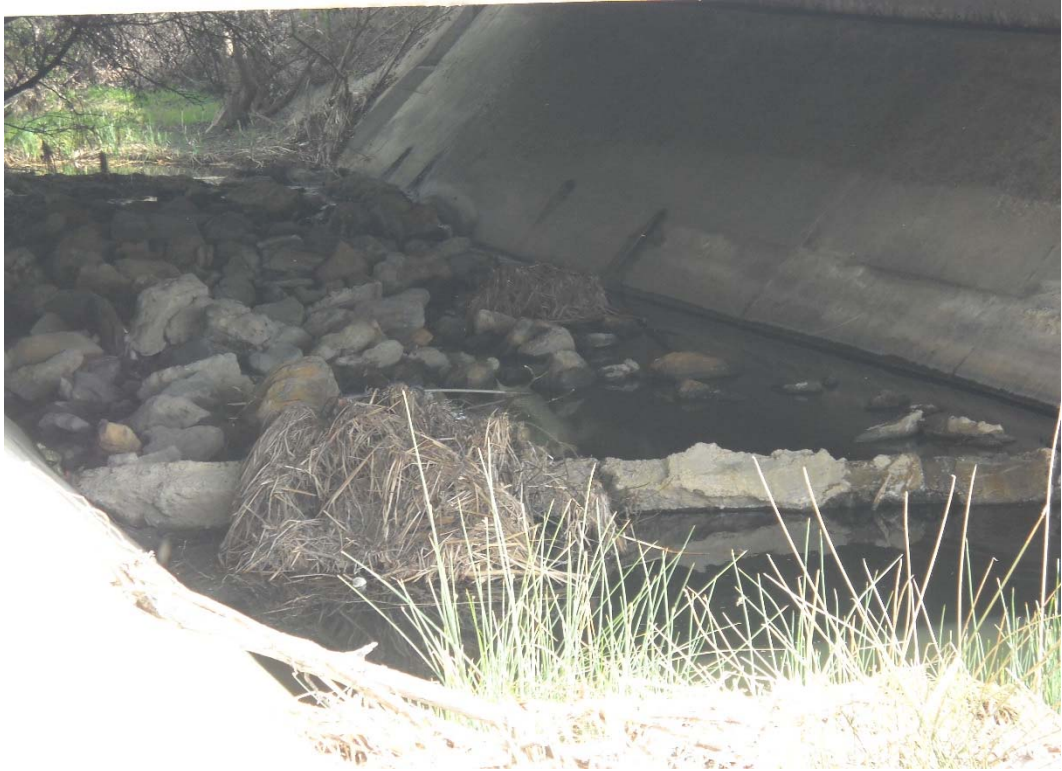
50 FT. UPSTREAM OF HEC-RAS RIVER STATION 58+85, UPSTREAM DIRECTION (BENEATH THOUSAND OAKS BLVD. BRIDGE)
