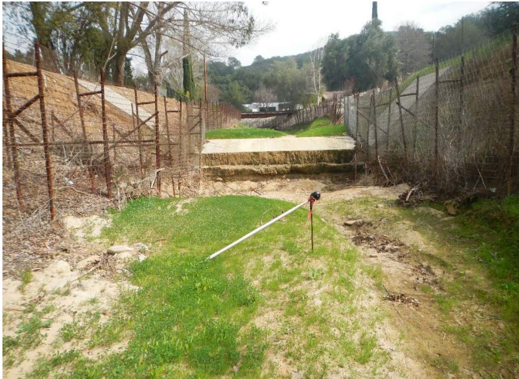
HEC-RAS RIVER STATION 19+06, UPSTREAM DIRECTION
