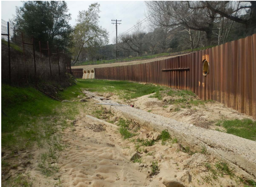
HEC-RAS RIVER STATION 17+54, DOWNSTREAM DIRECTION
