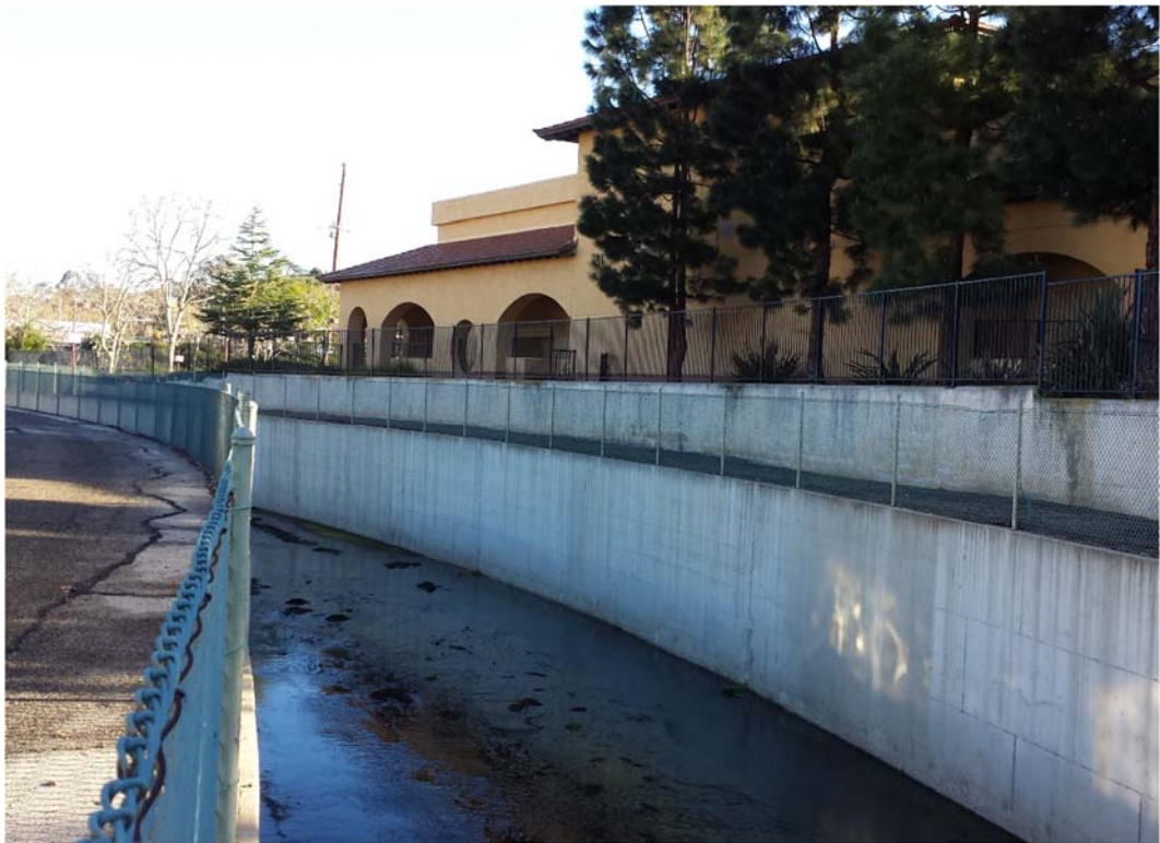
HEC-RAS RIVER STATION 17+34, UPSTREAM DIRECTION
