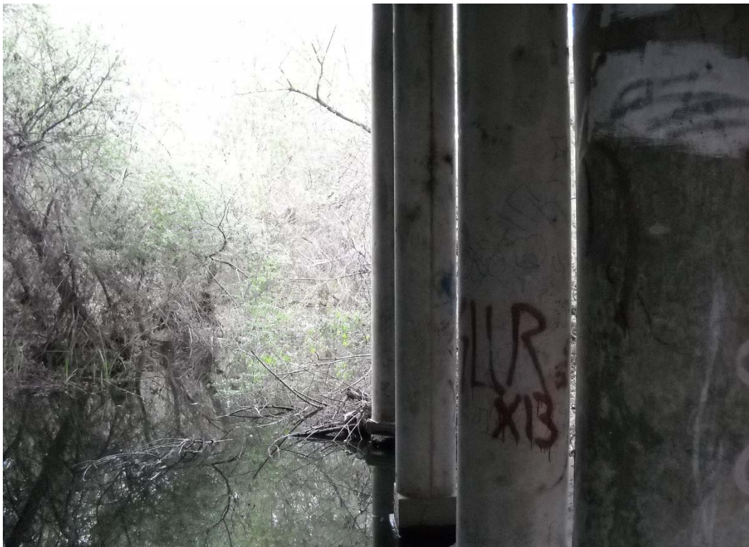
40 FT. UPSTREAM OF HEC-RAS RIVER STATION 25+35, UPSTREAM DIRECTION
