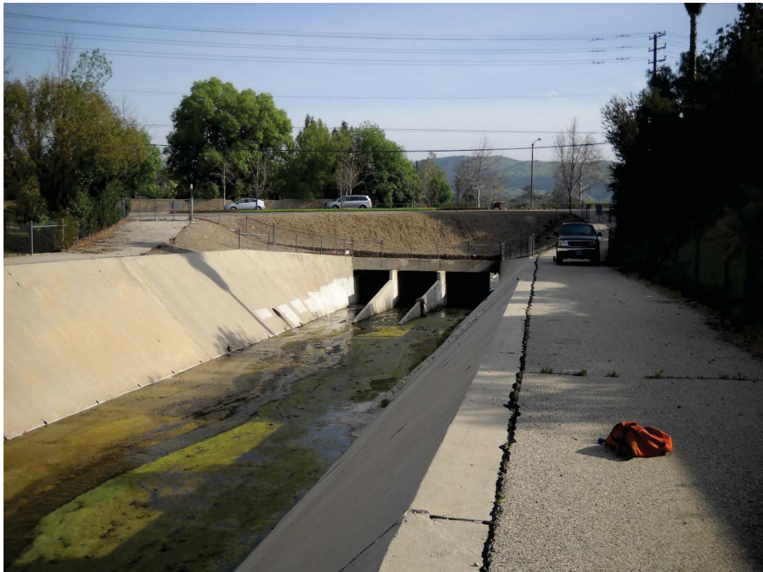
Figure 6-4. Box Culvert at Kanan Road
