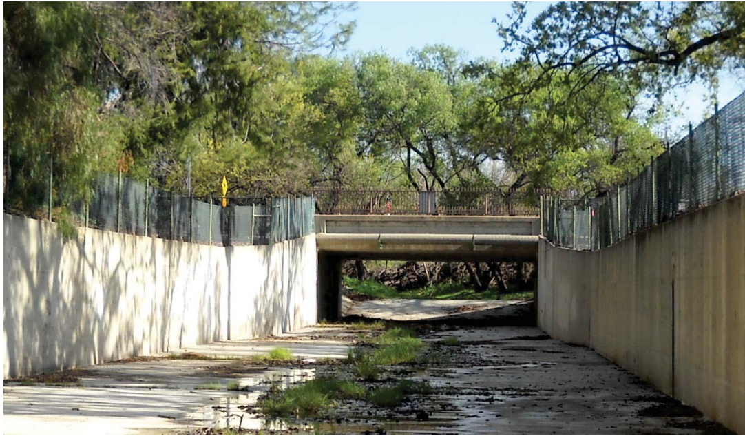
Figure 7-2. Driver Ave Culvert Downstream of Cheseboro Main Channel Inlet
