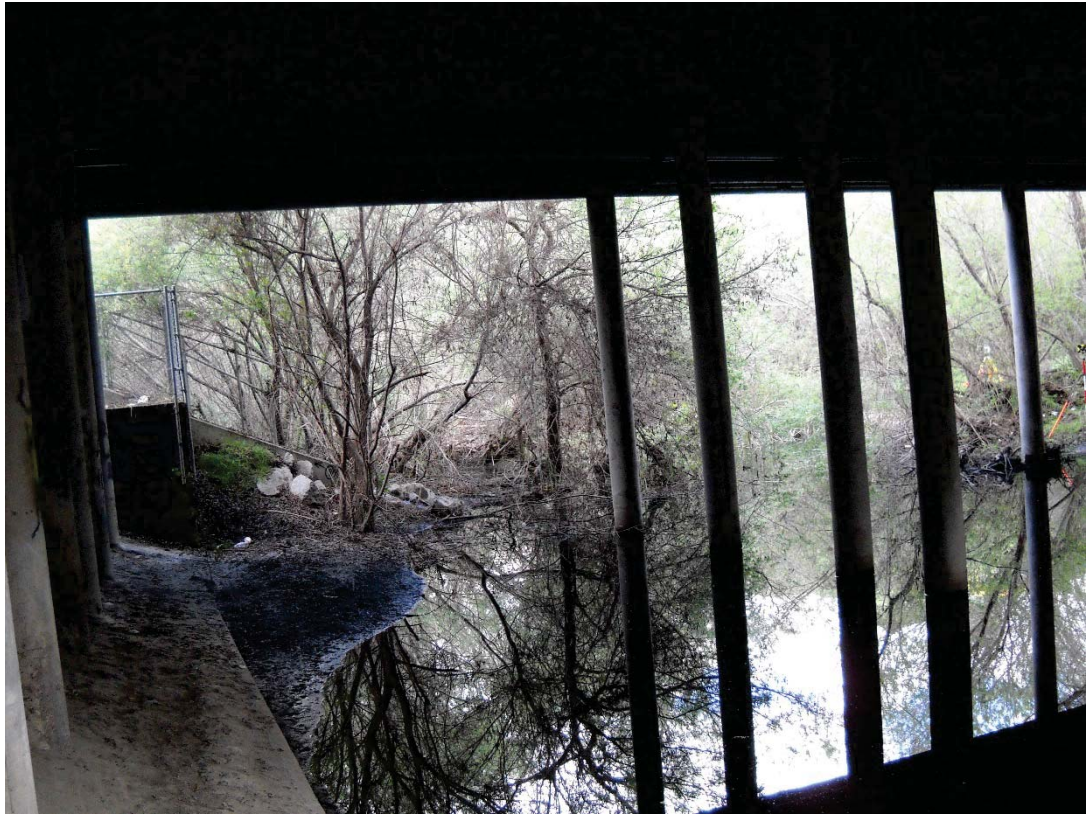
Figure 6-8. Beneath Canwood Street Bridge, Right Bank
