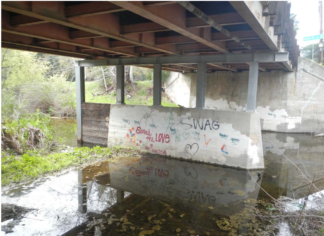
REACH DOWNSTREAM EXTENT, 83 FT. DOWNSTREAM OF HEC-RAS RIVER STATION 12+08, MULHOLLAND HIGHWAY BRIDGE
