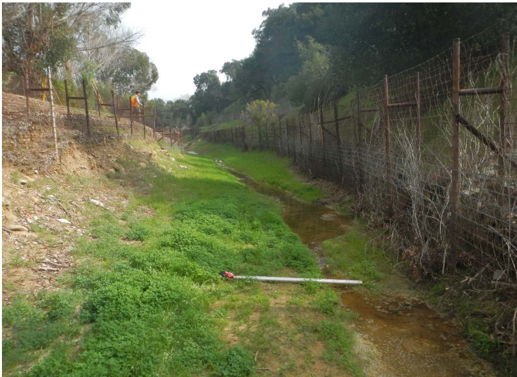
82 FT. UPSTREAM OF HEC-RAS RIVER STATION 21+08, UPSTREAM DIRECTION
