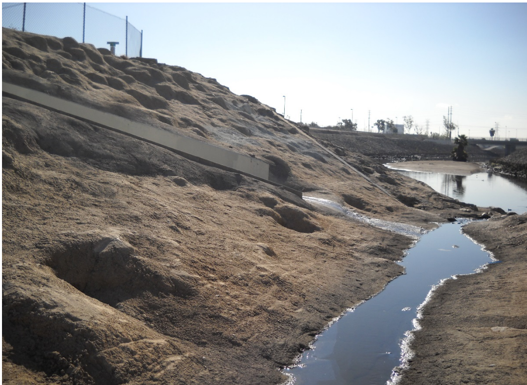
HEC-RAS RIVER STATION 01+01, DOWNSTREAM DIRECTION
