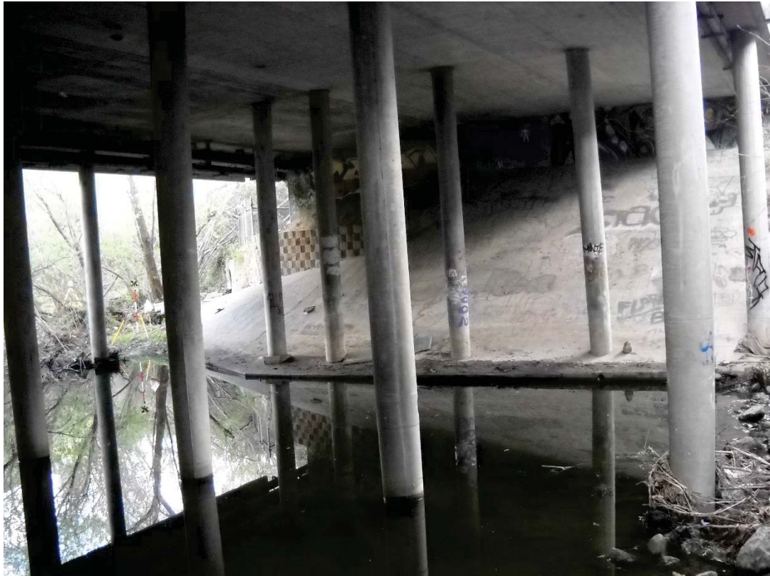
Figure 6-7. Beneath Canwood Street Bridge, Left Bank
