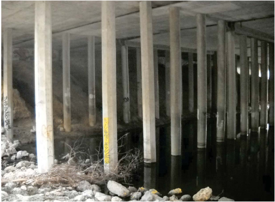
Figure 6-9. Beneath U.S. Highway 101 Bridge, Left Bank
