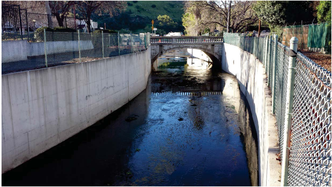
Figure 6-12. Agoura Road Bridge
