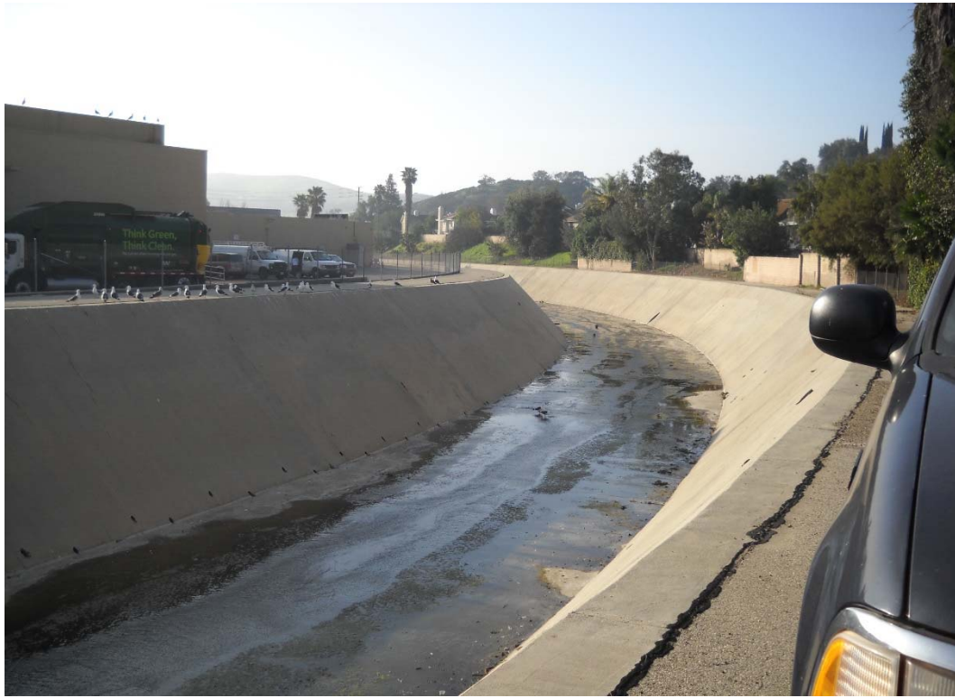
79 FT. DOWNSTREAM OF HEC-RAS RIVER STATION 57+19, DOWNSTREAM DIRECTION (DOWNSTREAM OF REACH NO. 33)
