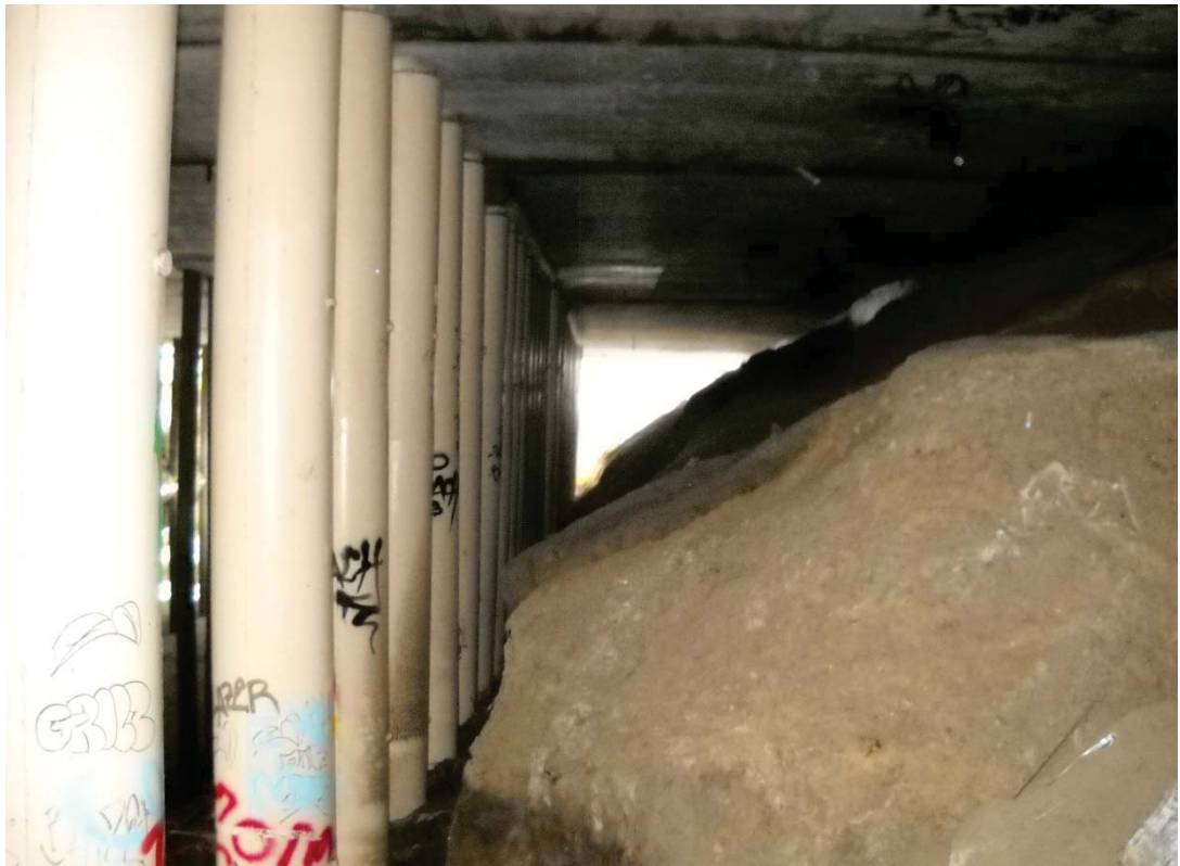
Figure 6-10. Beneath U.S. Highway 101 Bridge, Right Bank
