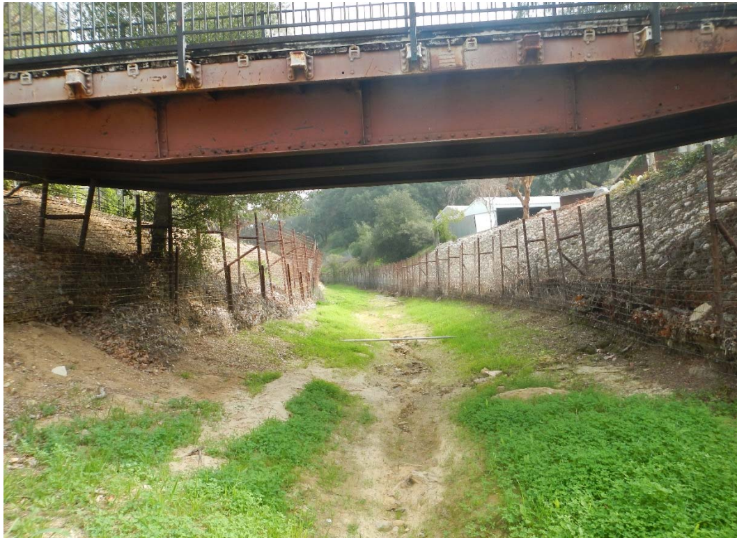
HEC-RAS RIVER STATION 21+08, UPSTREAM DIRECTION (PRIVATE DRIVEWAY BRIDGE)
