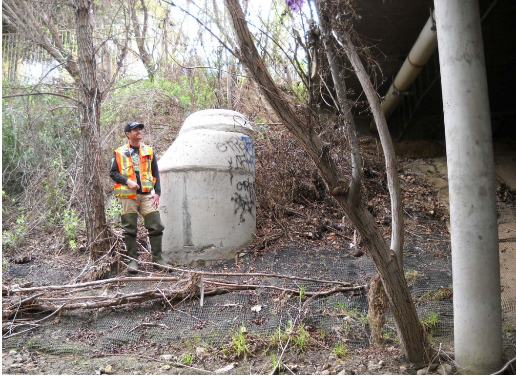
HEC-RAS RIVER STATION 32+12, RIGHT BANK (DOWNSTREAM OF OAK CREEK LN. BRIDGE)
