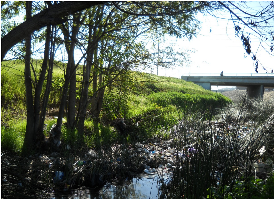
HEC-RAS RIVER STATION 3+70, DOWNSTREAM DIRECTION
