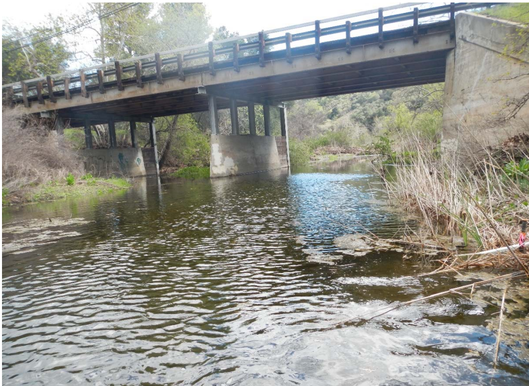
HEC-RAS RIVER STATION 12+08, DOWNSTREAM DIRECTION (MULHOLLAND HWY BRIDGE)
