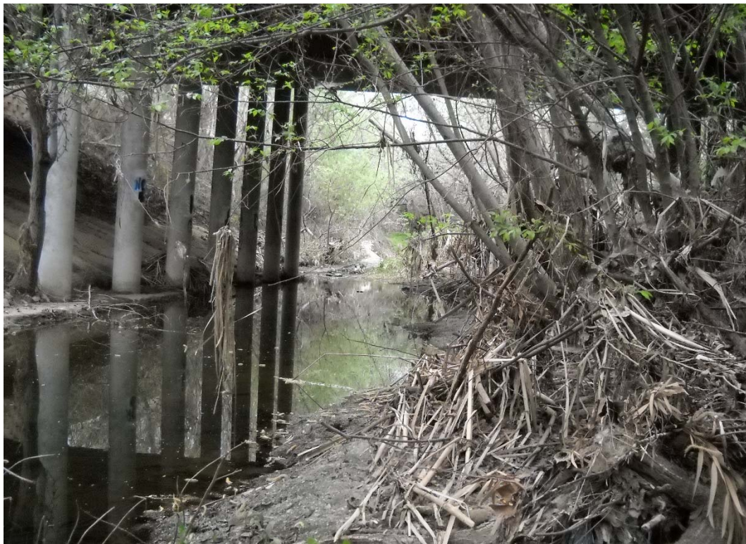
HEC-RAS RIVER STATION 31+89, UPSTREAM DIRECTION (OAK CREEK LN. BRIDGE)
