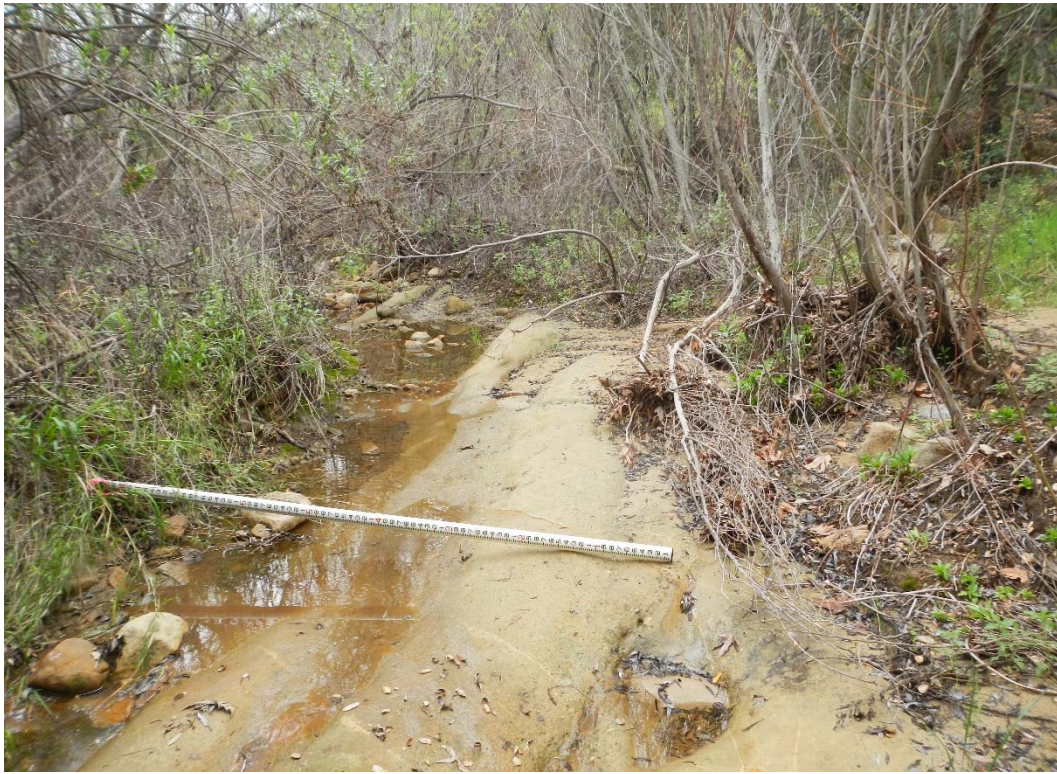
HEC-RAS RIVER STATION 32+64, UPSTREAM DIRECTION
