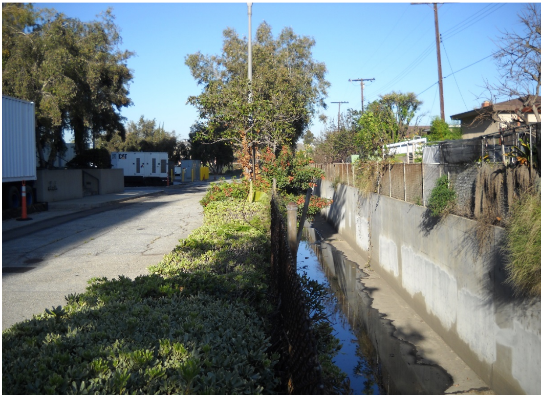
HEC-RAS RIVER STATION 13+50, UPSTREAM DIRECTION
